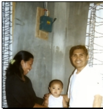
Fuse box for new electric service
